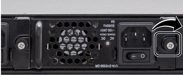
Figure 2-7 Installing the Power Module
