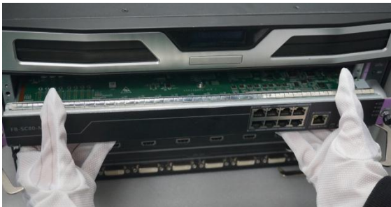
Figure 2-2 Installing the Control Board and Service Boards
